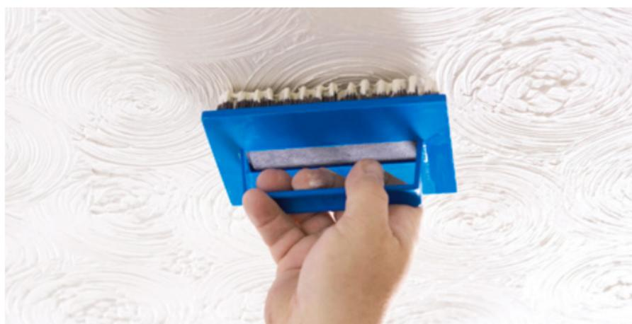
Continue in this way, completing successive bands until the whole area is finished. Work quickly but carefully to make sure bands can be blended while the material is still wet.
