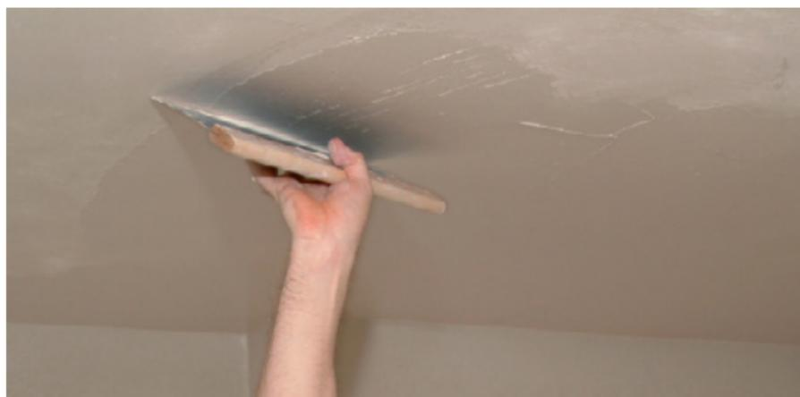
When dry, minor imperfections can be lightly sanded. Remove any dust before applying a final liberal coat of Artex Stabilex.
