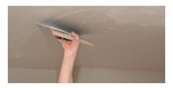
When dry, minor imperfections can be lightly sanded. Remove any dust before applying a final liberal coat of Artex Stabilex.
